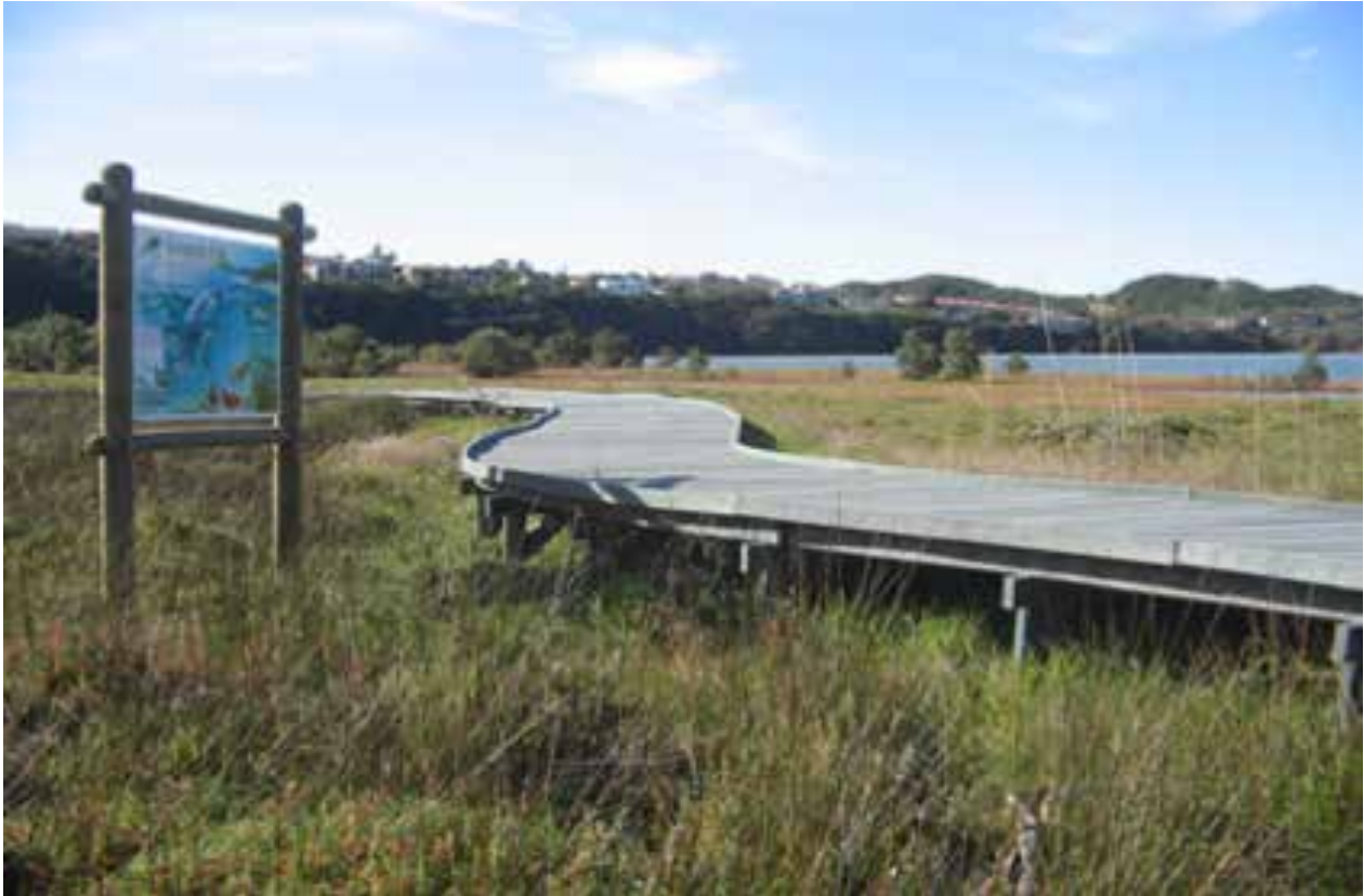
Plate 8: Upgraded boardwalk at Nahoon Estuary Reserve
