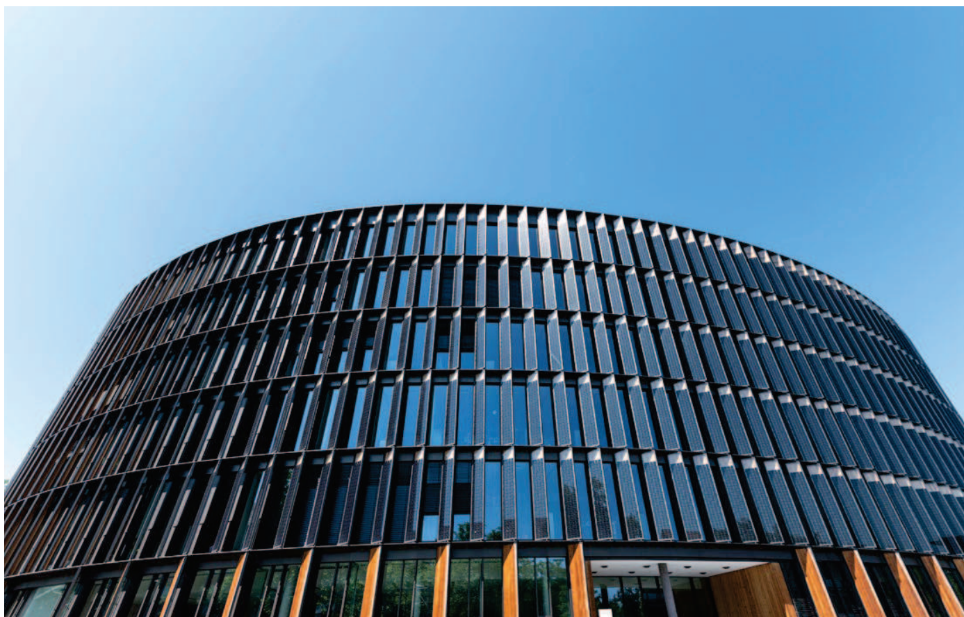
Photo 16: The facade of the town hall in Stühlinger covered with photovoltaics. © Stadt Freiburg, Amt für Bürgerservice
