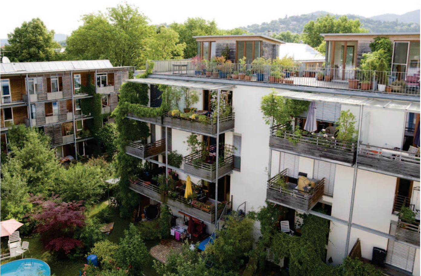
Photo 24: Green residential buildings in the Freiburg district of Vauban © FWTM, Schoenen
