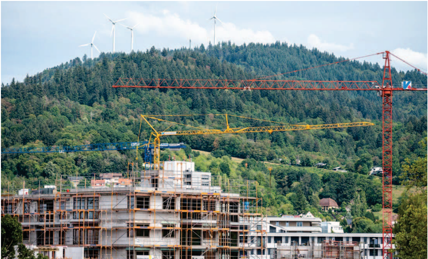
Photo 22: A construction site in Freiburg © Stadt Freiburg
