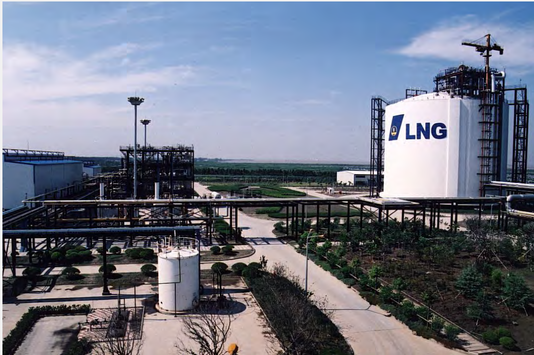
Figure 11 LNG Terminal in Wuhaogou, Pudong New Area
