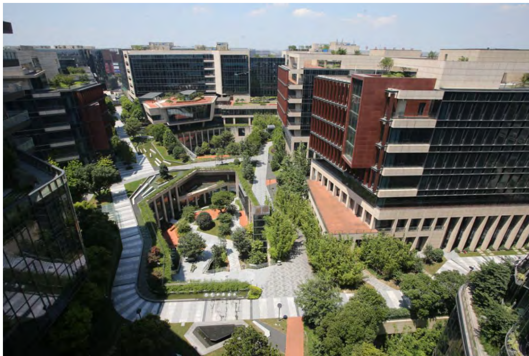
Figure 26 Hongqiao Green Valley Plaza
