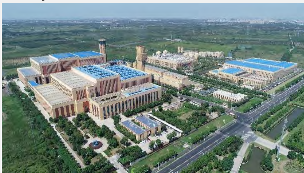
Figure 25 Incineration Plant in Tianma Zero-waste Low-carbon Eco-friendly Industrial Park in Songjiang District
