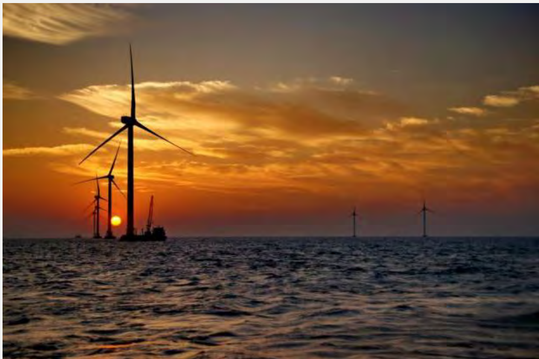
Figure 10 Offshore Wind Farm near Donghai Bridge, Shanghai
