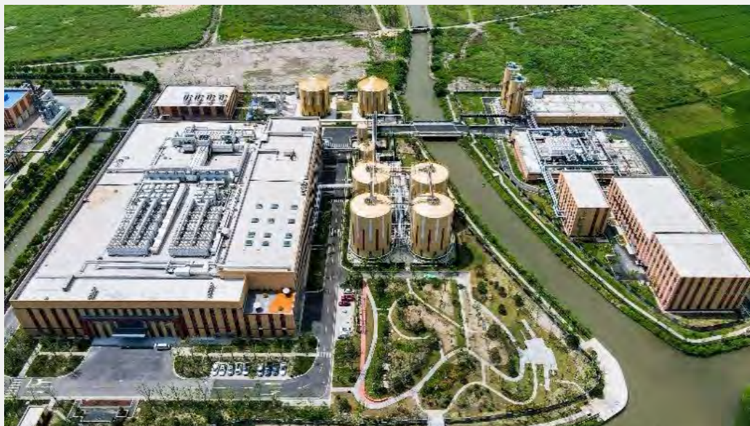
Figure 17 Wet Waste Incineration Plant of Tianma Zero-waste Low-carbon Environmental Protection Industrial Park
