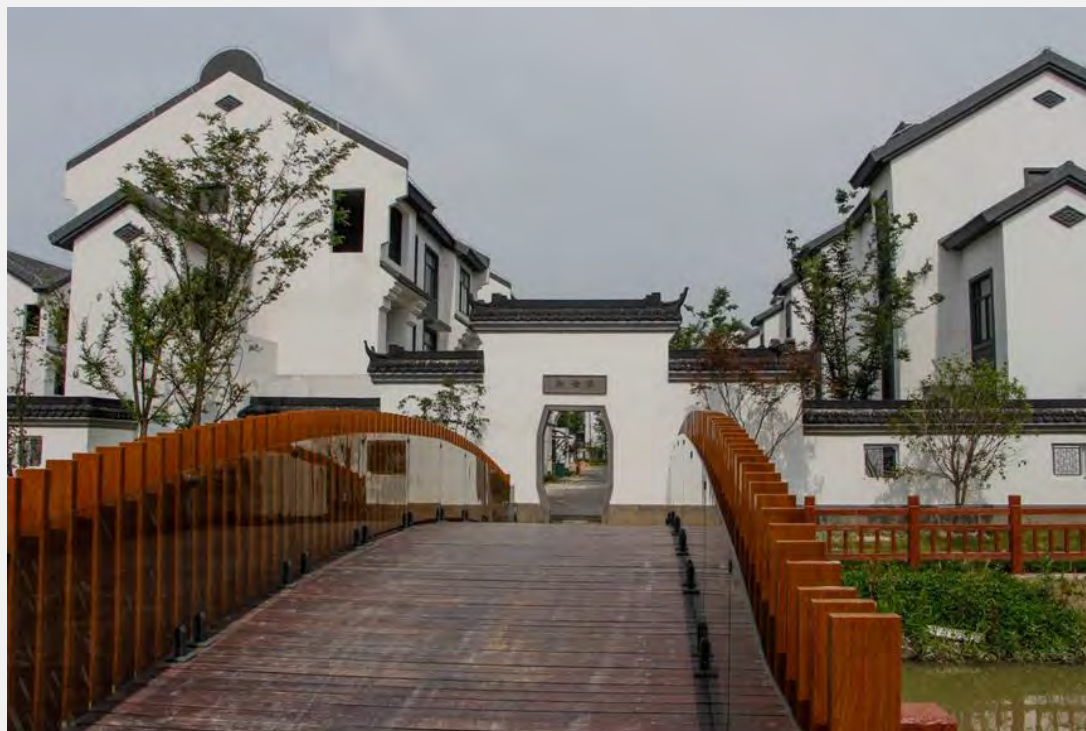
Figure 15 Village Appearance after Rectification
