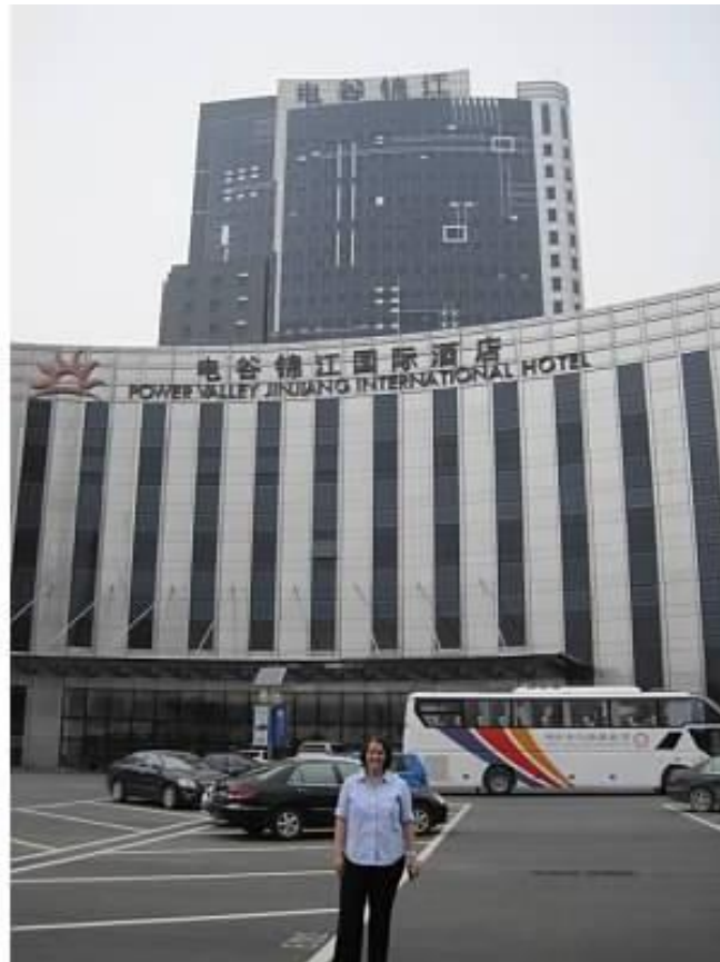
Photo of Building Integrated PV hotel in Baoding, China
