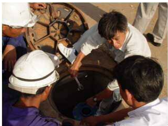
Water supply project at Phnom Penh
