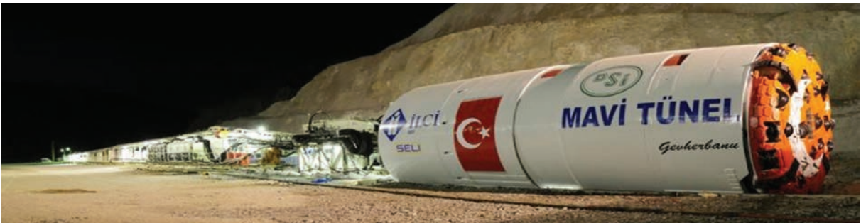
Photo: Konya Blue Tunnel drinking water project
