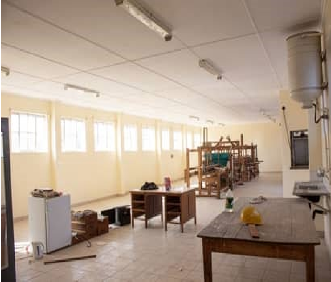
Project paintwork and tiling . Carport complete
