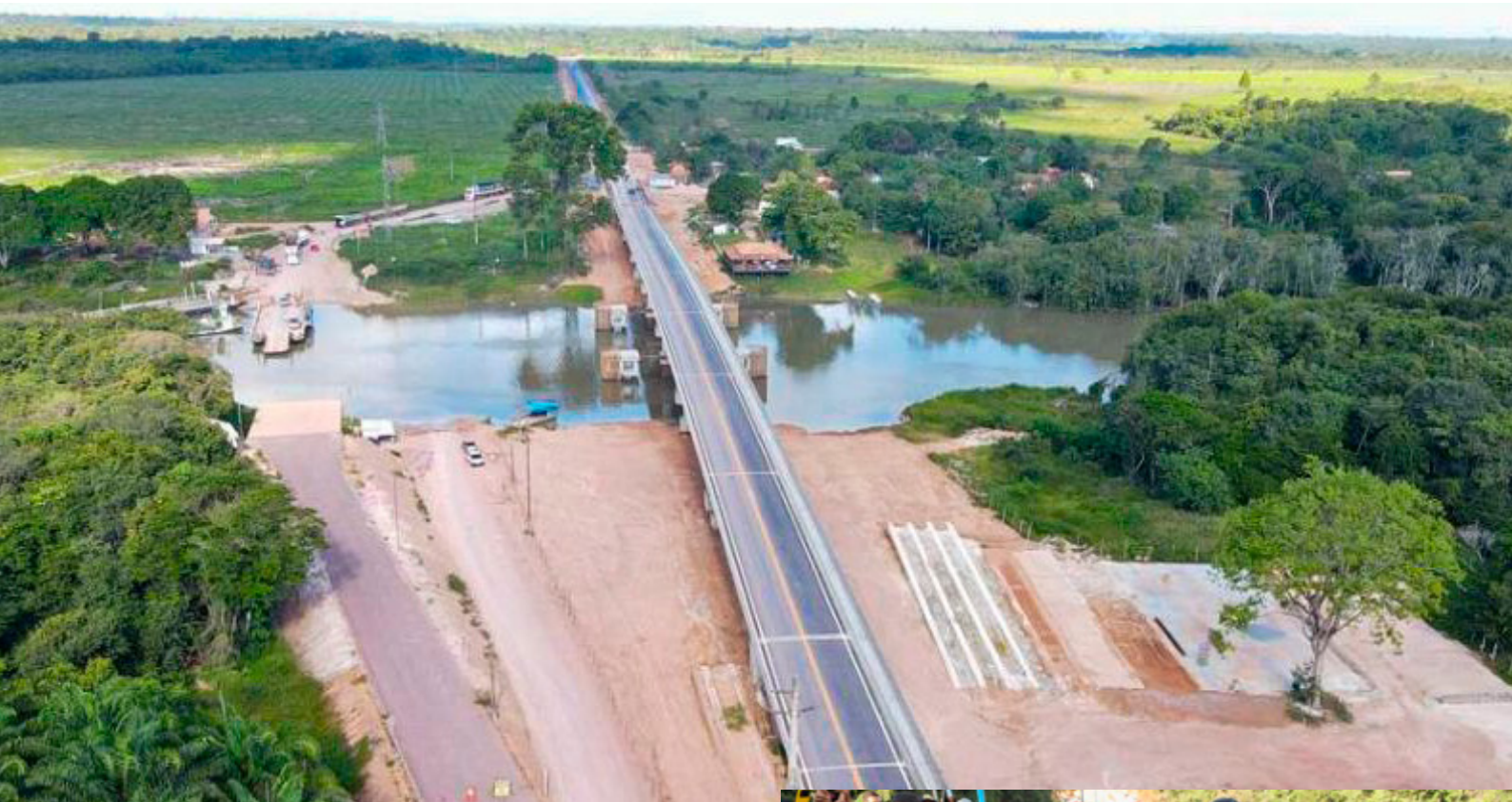
Bridge over the Alto Acará River
