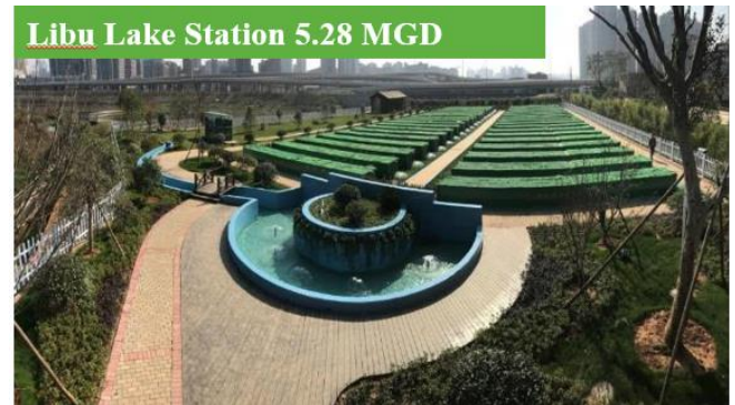
Figure 4. Libu Lake FMBR wastewater treatment plant site
