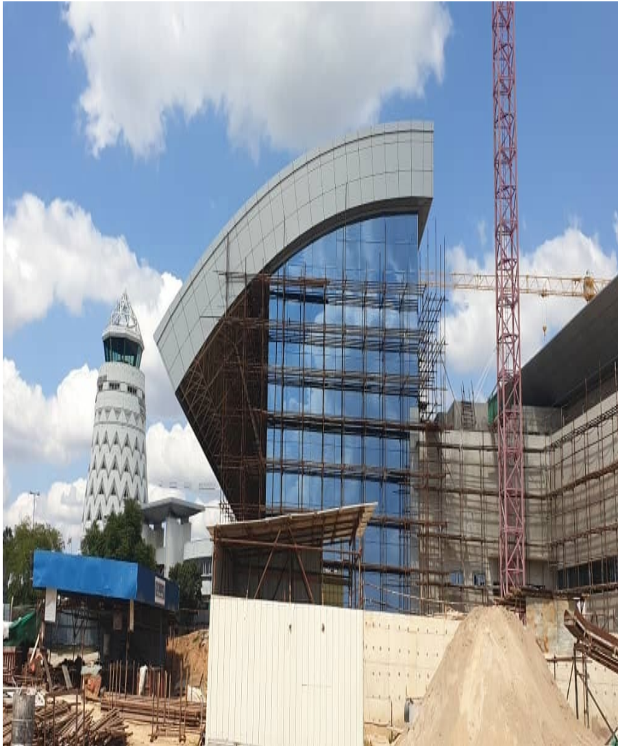
Outside of Terminal Building (72% Complete)
