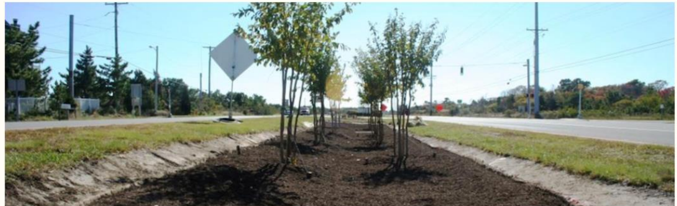
Storm water retrofits prevent water from washing into storm drains, allowing it to soak and filter into the ground.
