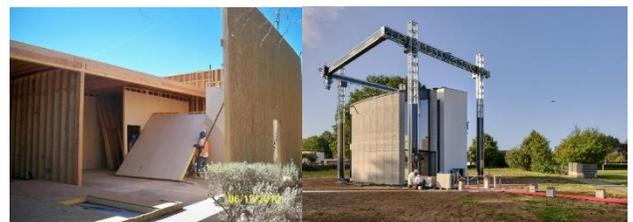
Combining the two technologies into M3DP marries the customizability, cost-efficiency, and on-site construction of 3DP houses with the adjustable qualities of modular construction. M3DP entails that the modules of the house are printed and assembled on-site. Figure A1 shows a schematic representation of the combination of modular construction and 3DP construction into M3DP. M3DP could contribute to the construction of adjustable, affordable, and climate-resilient houses.
