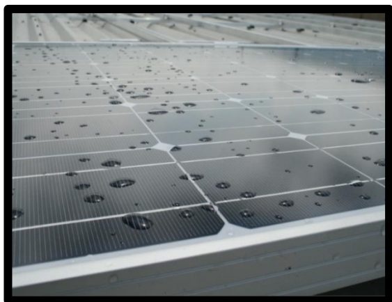
Figure 4. Hydrophobic coating applied to solar panels
