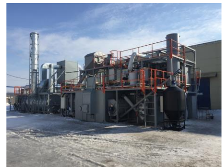
Figure 2. Germany Plant Reactor. Copyright 2020 Biogas Energy Inc.
